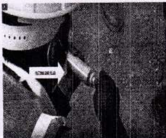
Fixing end plug to attach Chinese finger
